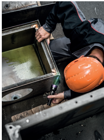
Dye penetrant testing
